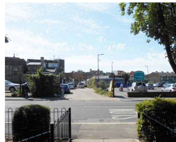
Shared vehicular access road
