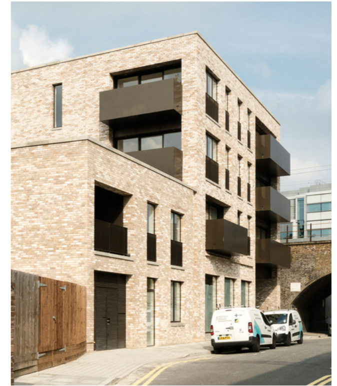
Light buff brick with metal projecting balconies. Karakusevic and Carson. Great Eastern Buildings.
