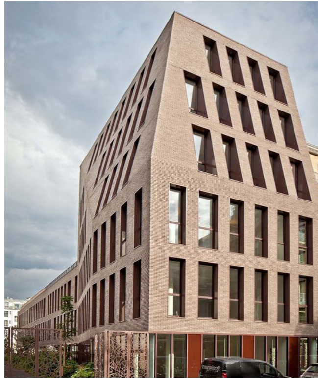
Slanted facade, full height windows and deep reveals
