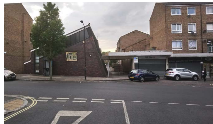
1. View from Oswyth Road
