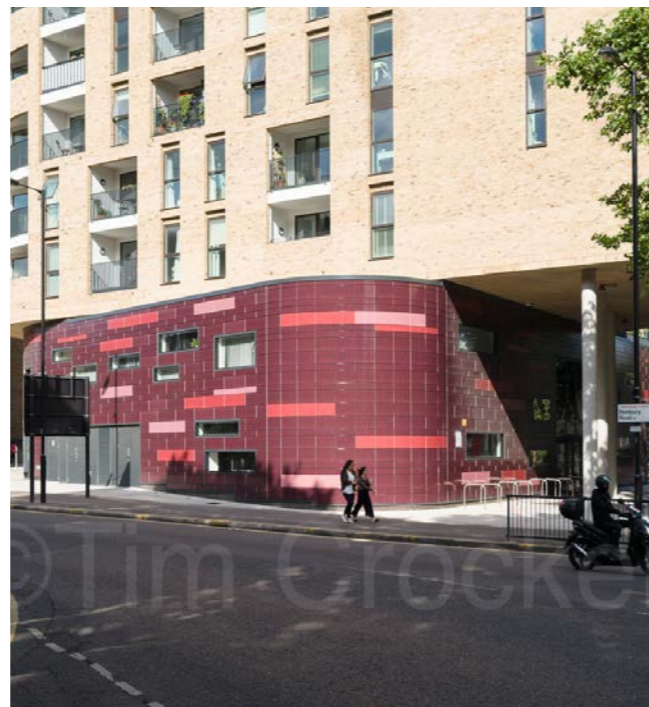
Clear difference between building uses in terms of materials and shape. FBM Architects. Pembury Circus
