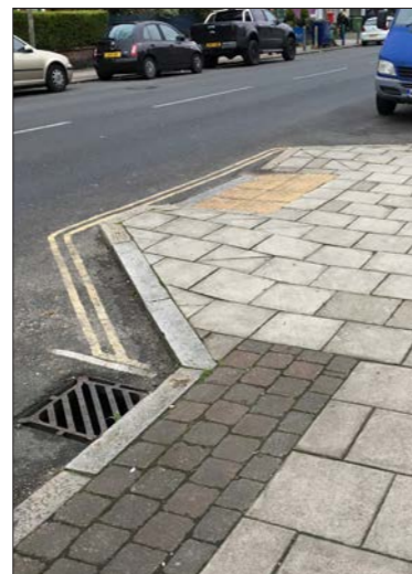
Typical road crossing
