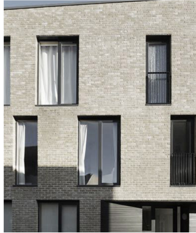
Full height windows with dark frames and reveals
