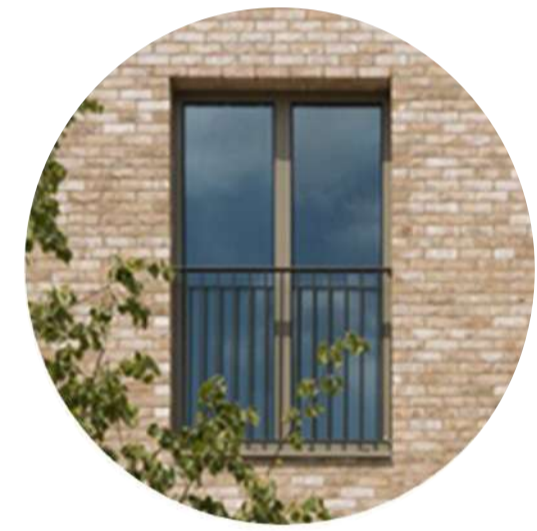
Powder coated window frames, metal balustrade and reveals, colour warm grey
