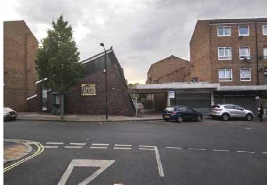
1 View from Oswyth Road to the site.
