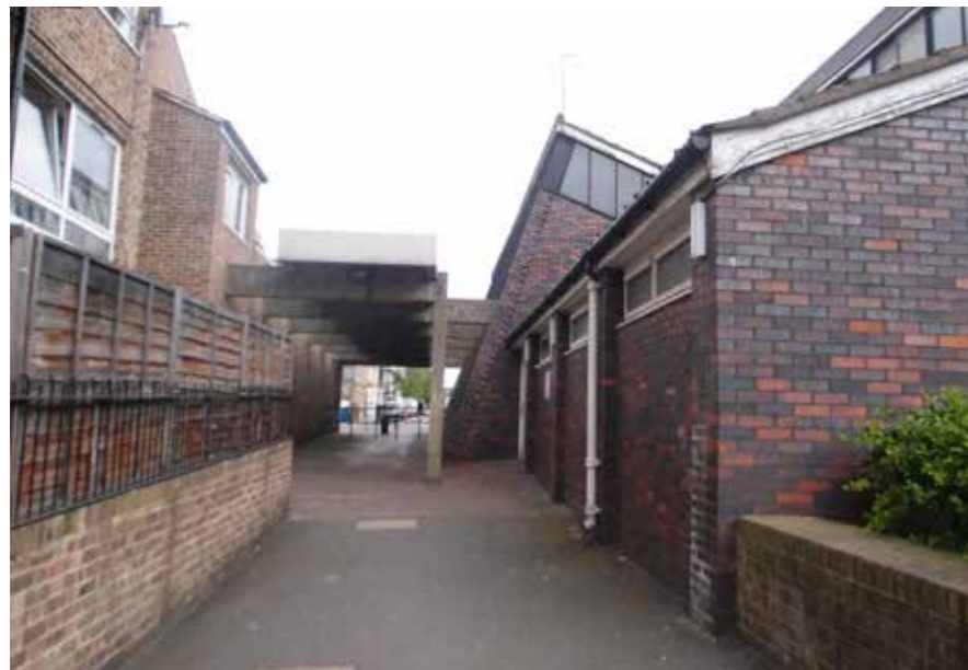
3 Pathway on the north of the site.
