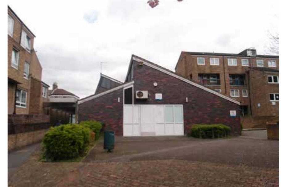
2 View from the community garden of Pembury House
