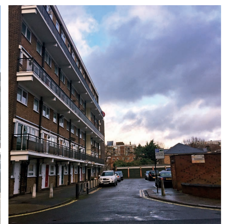
4. Access road from Grange Walk
