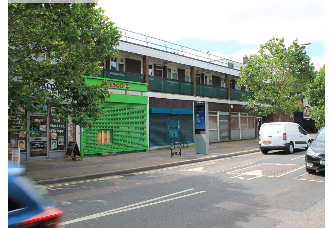
2. Existing building from Rotherhithe New Road
