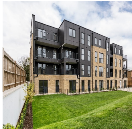
Milton House, Croydon
