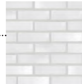
White glazed Brick, white mortar to walls within 'lightwell'
