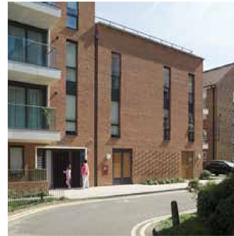
Masterman House garages / Lomond Grove SE5
