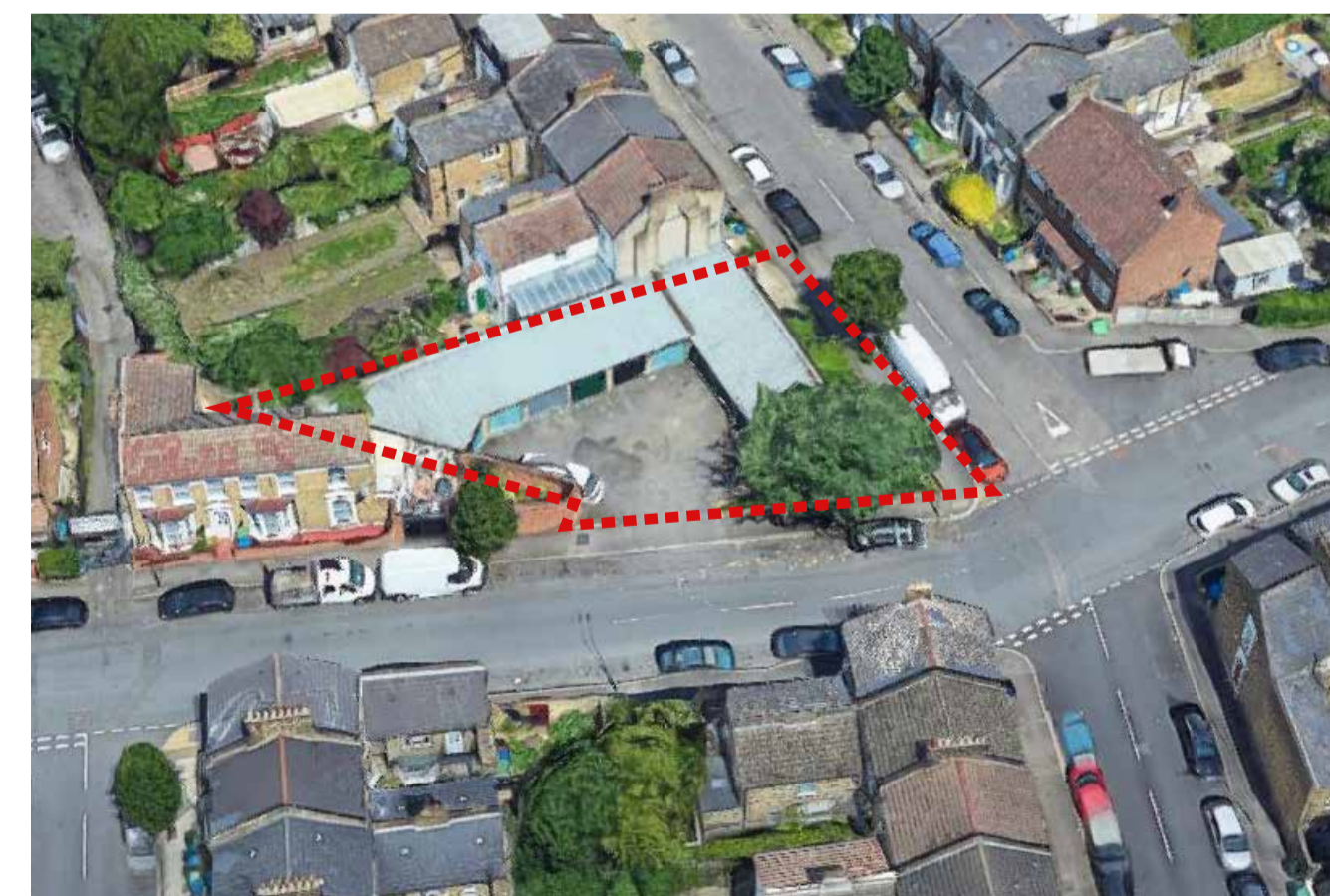
4. Aerial view to the site
