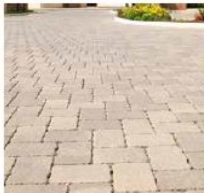
Permeable paving to the entry area. Permeable paving to allow for irigation of the tree roots. Colour- light buff
