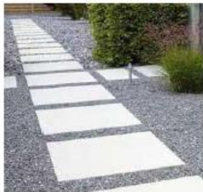
Pavers to defensive space- access for maintenance.
