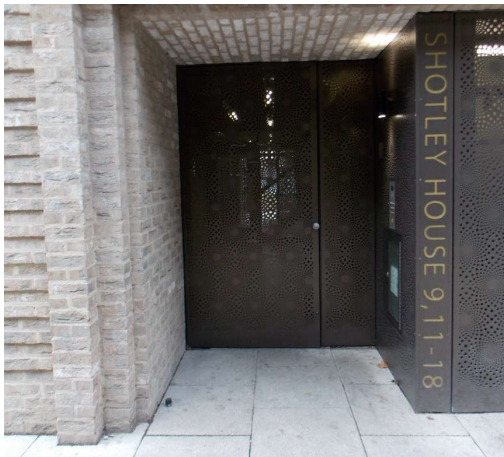
Bins neatly concealed
