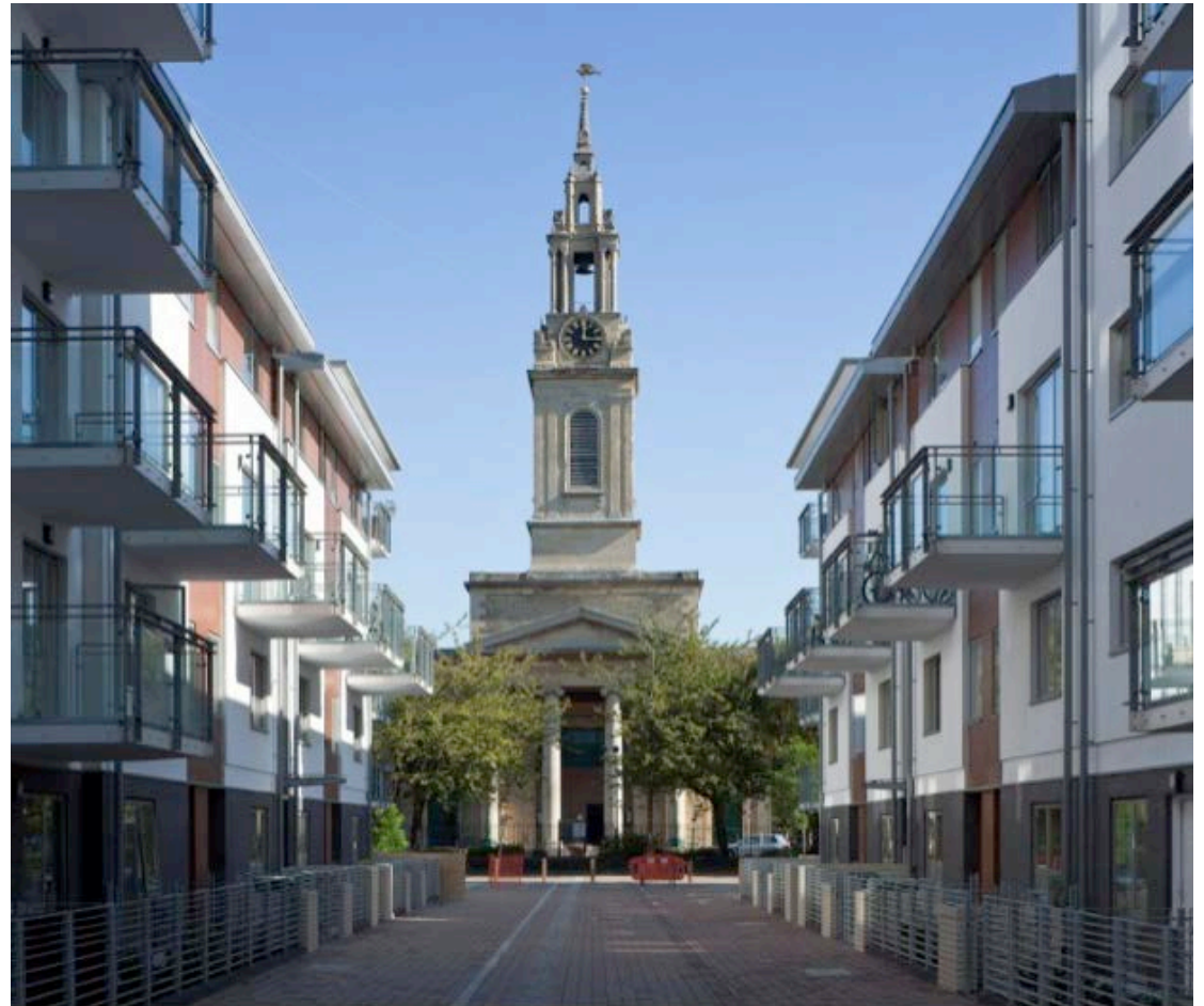
New pedestrian street, Bermondsey Spa regeneration
