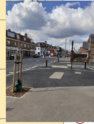
Existing widened footway in temporary materials to be replaced with permanent materials
