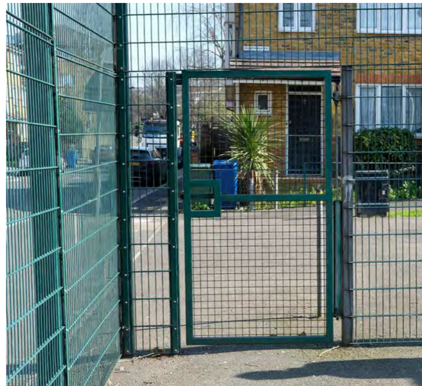
Fencing inhibits access
