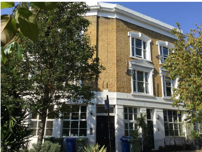
Figure 21 The Globe former public house, Darwin Street
