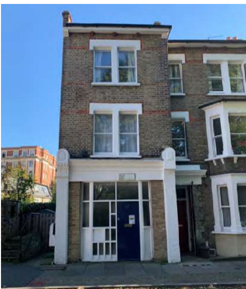
Figure 41 No. 67 Balfour Street with former shopfront
