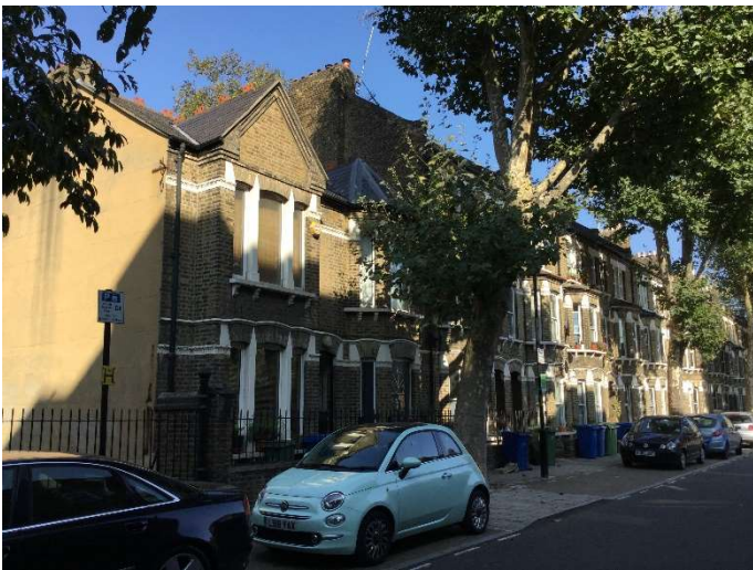
Figure 34 Nos 13–26 Searles Road
