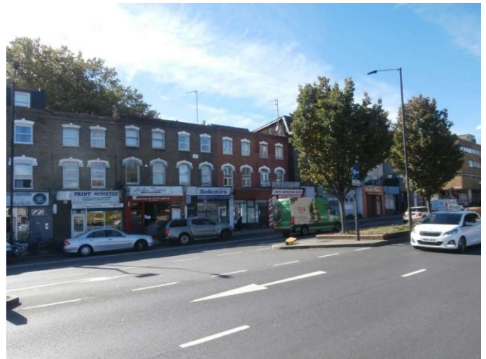
Figure 2 Nos 620–636 Old Kent Road
