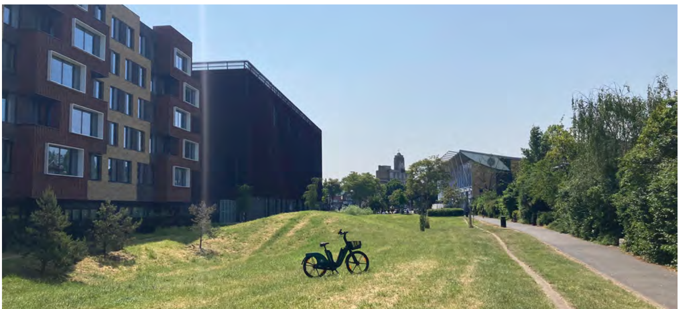
UAL student accommodation and the Mountview Academy building.
