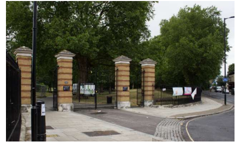
China Hall Gate
