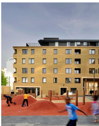
Peabody Avenue, Pimlico: A courtyard housing project with play space.
