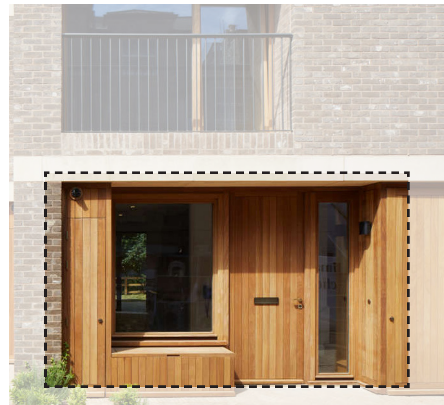
Built in 'street clutter' by front door
