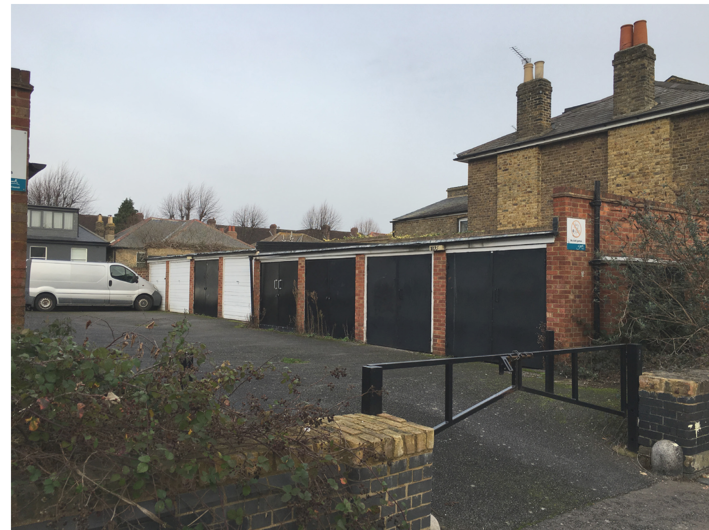
Garage site - flank wall from victorian terrace to the North
