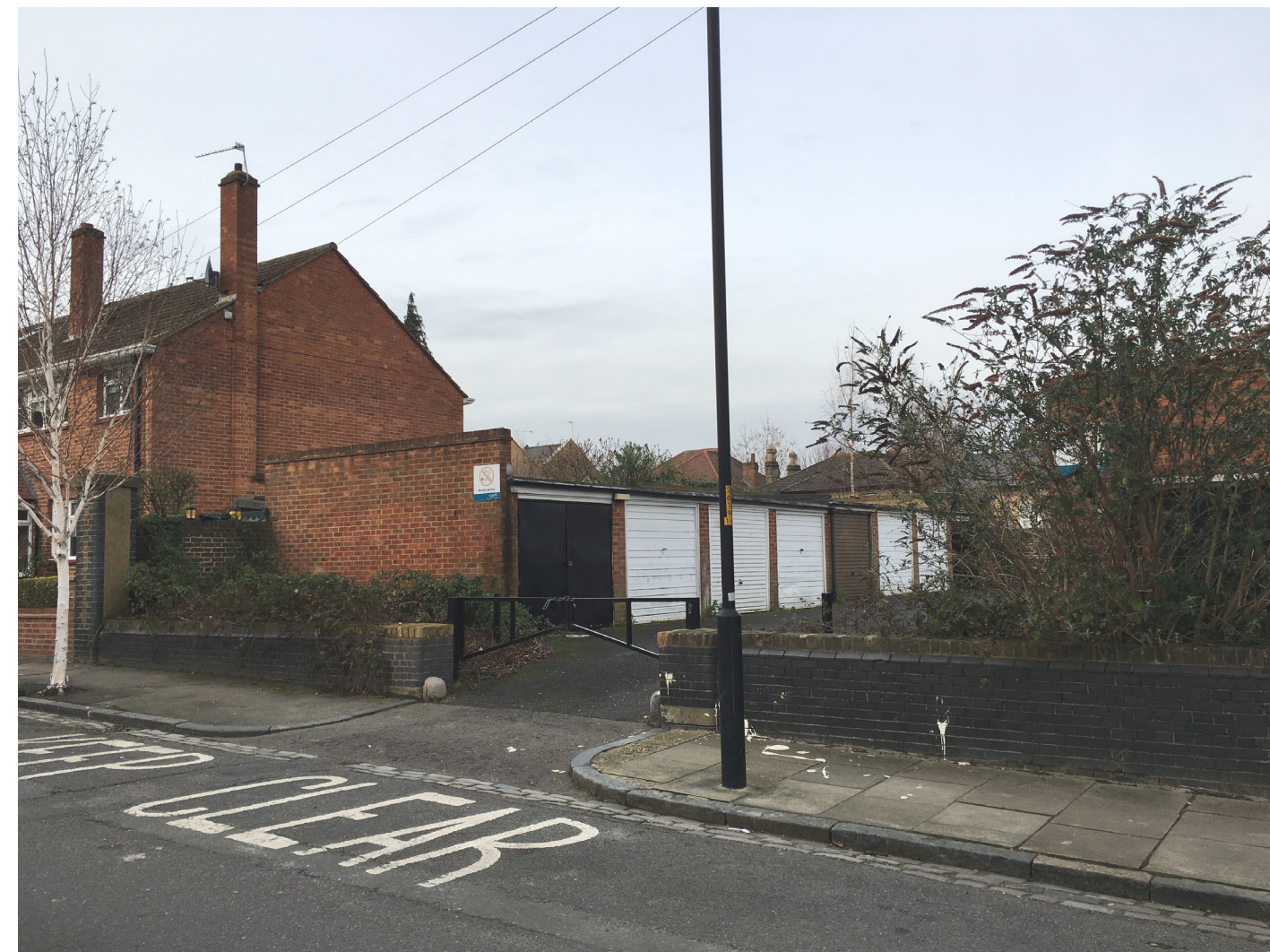
Garage site - flank wall of home to the South
